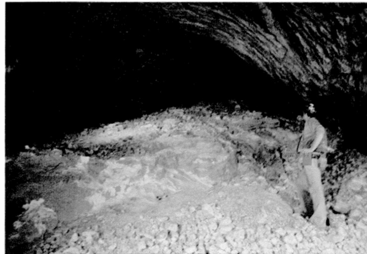
1975 blowout in 7 Main Entry West Room 4.
